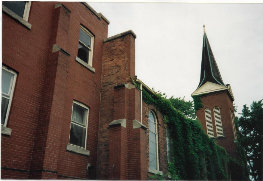
EAST FAÇADE, TOWER + SPIRE
