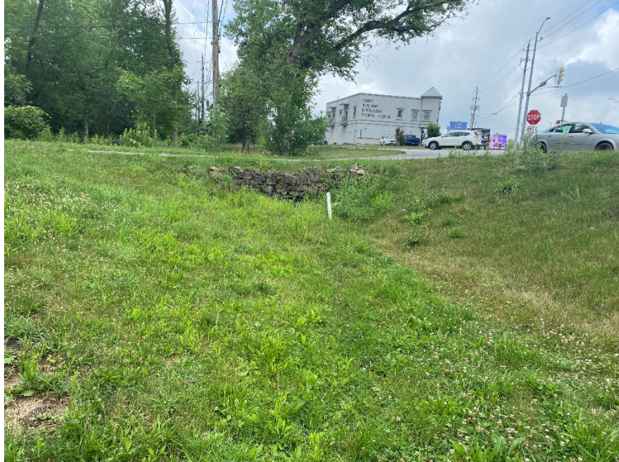
Photo 7: Facing south, H1-R2 (07-09-2021).
