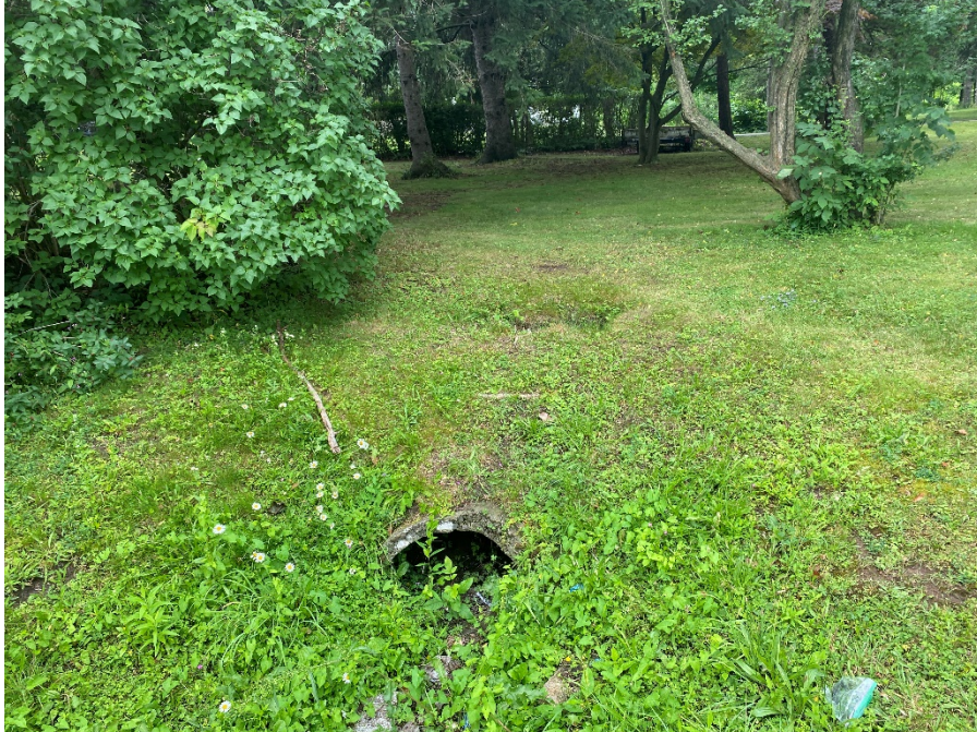
Photo 3: Facing south, H1-R6 (07-09-2021).
