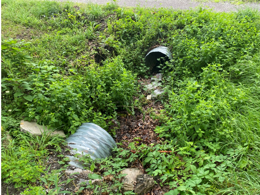
Photo 5: Facing south, H1-R4 (07-09-2021).
