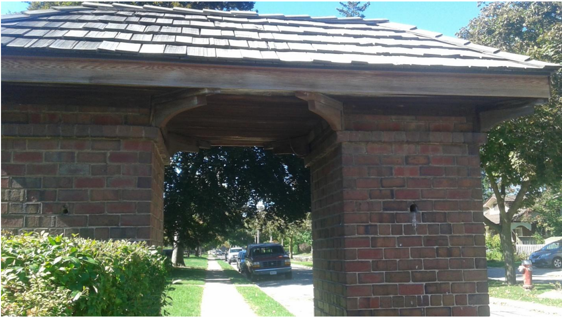
Figure 5 South archway Photo N. Reid Oct. 8, 2016
