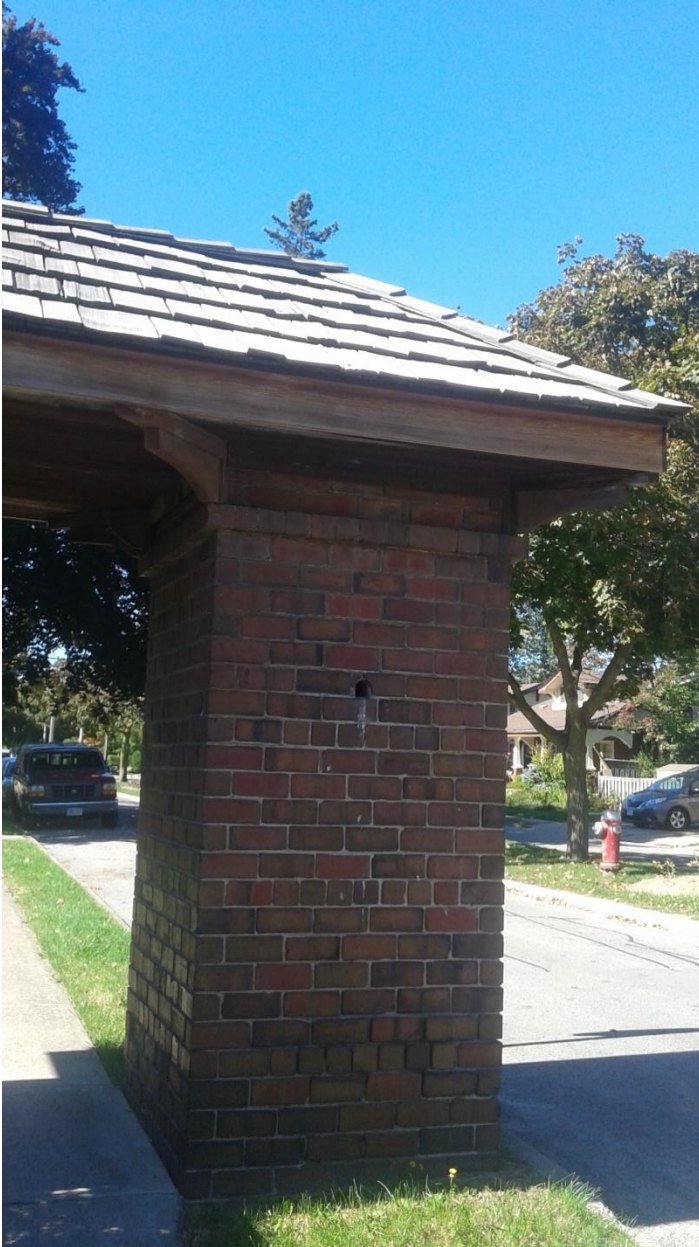
Figure 7. South archway. Photo N. Reid Oct. 8, 2016
