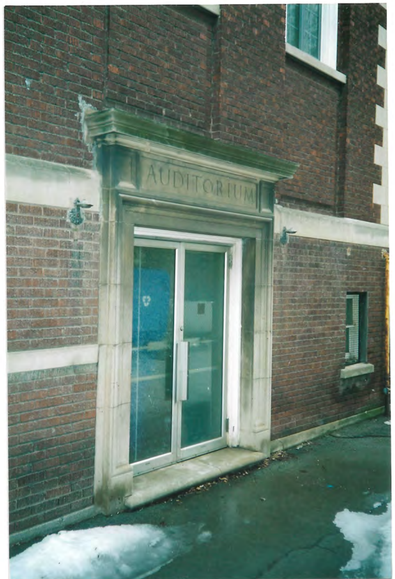
Figures 18 & 19 Welland Public Library, south facade with auditorium entrance at basement level
