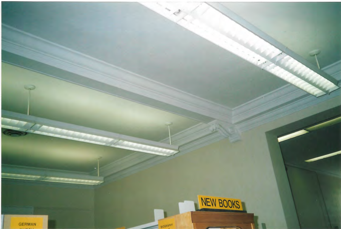
Figure 31 Welland Public Library Ceiling, original library
