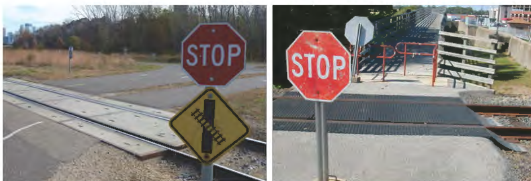
Photo: Track Crossing Material Alternatives to Asphalt (Left: Concrete) (Right: Rubberized Matting)
