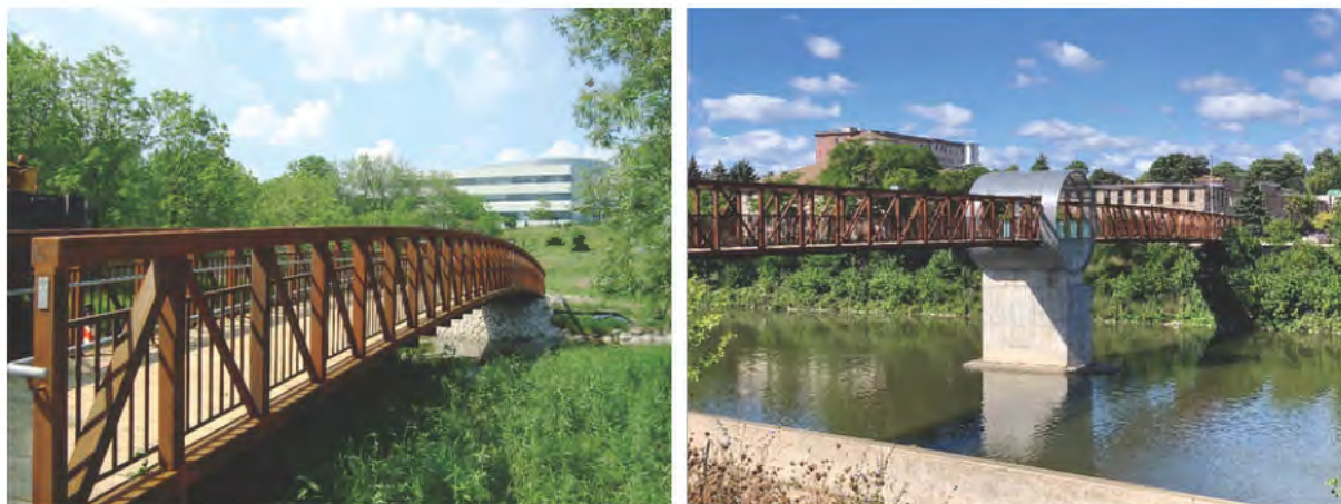
Photos of Pedestrian Bridges (Left: Etobicoke Creek Trail, 35+/-m)+ (Right: Craig's Crossing in Galt, two sections 55m+/- long)
