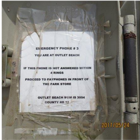
Existing script in emergency phone box
