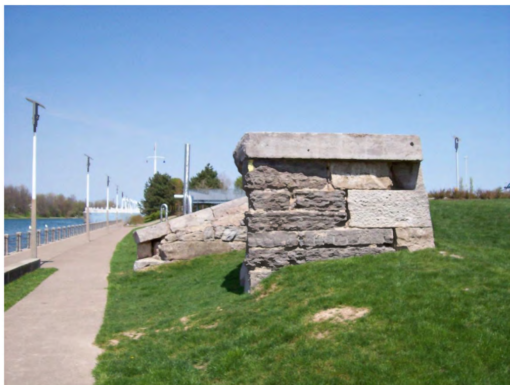
Fig. 23 & 24 Second Canal Aqueduct 2007
