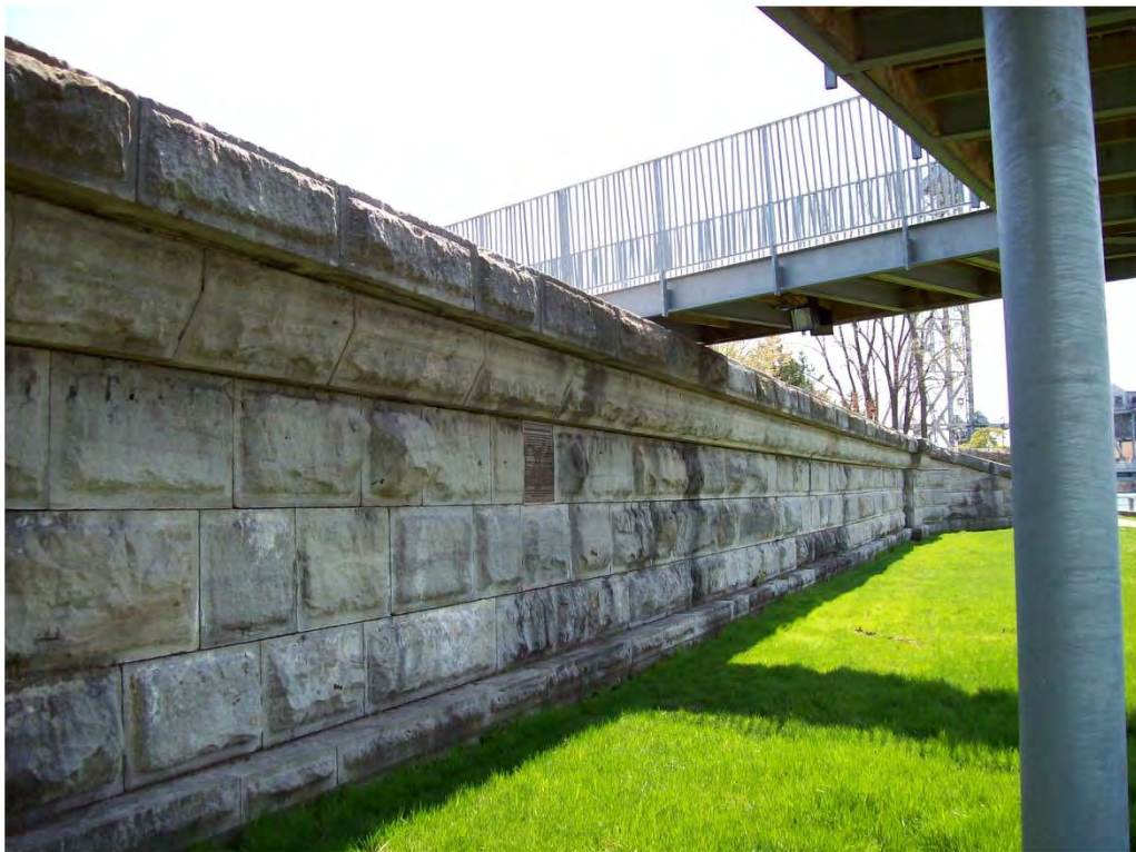
Figs. 15 & 16 Second Canal Aqueduct 2007
