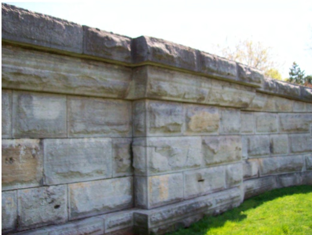
Figs. 19 & 20 Second Canal Aqueduct 2007
