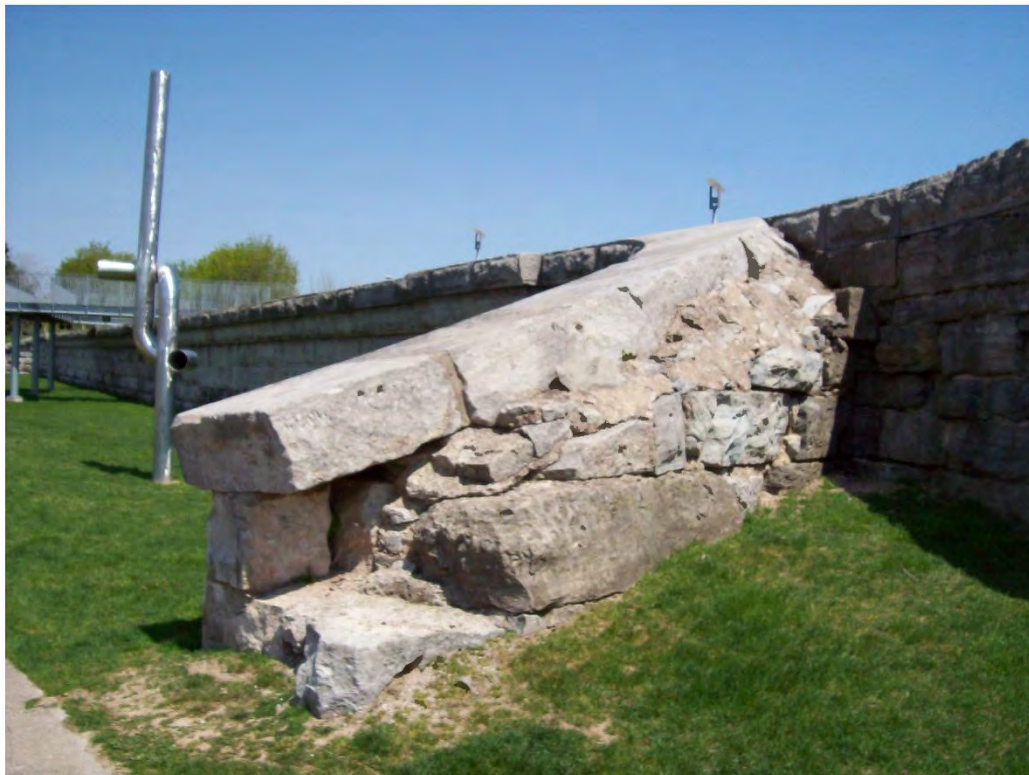
Figs. 21 & 22 Second Canal Aqueduct 2007
