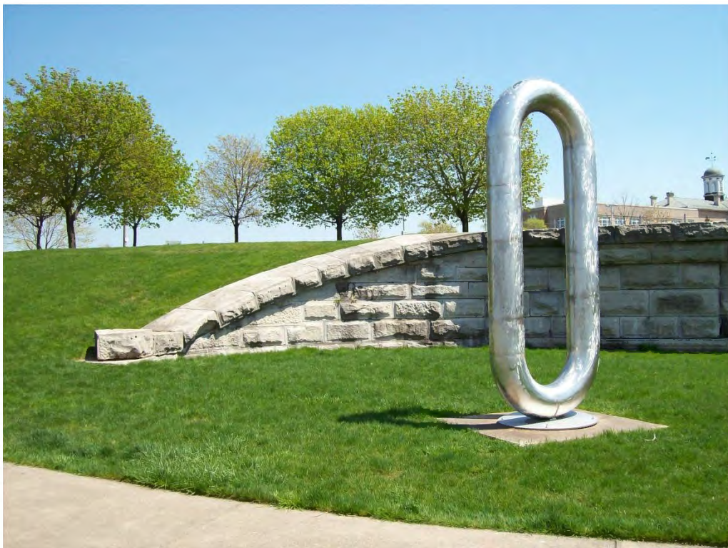
Figs. 11 & 12 Second Canal Aqueduct 2007
