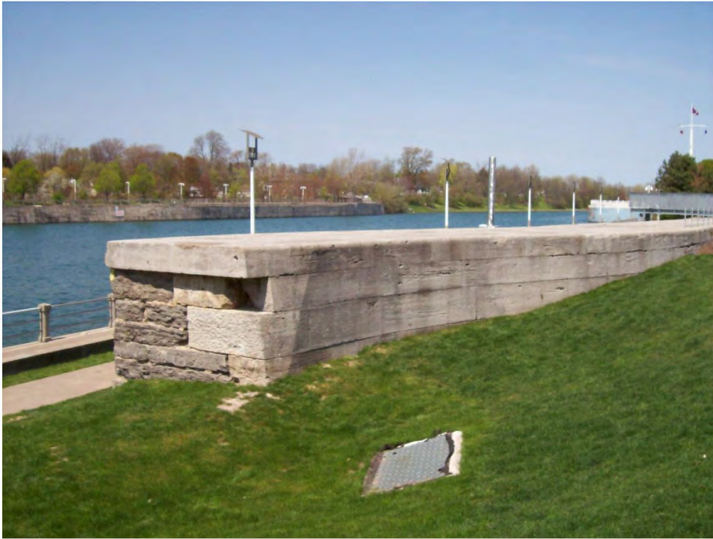
Fig. 25 Second Canal Aqueduct 2007
