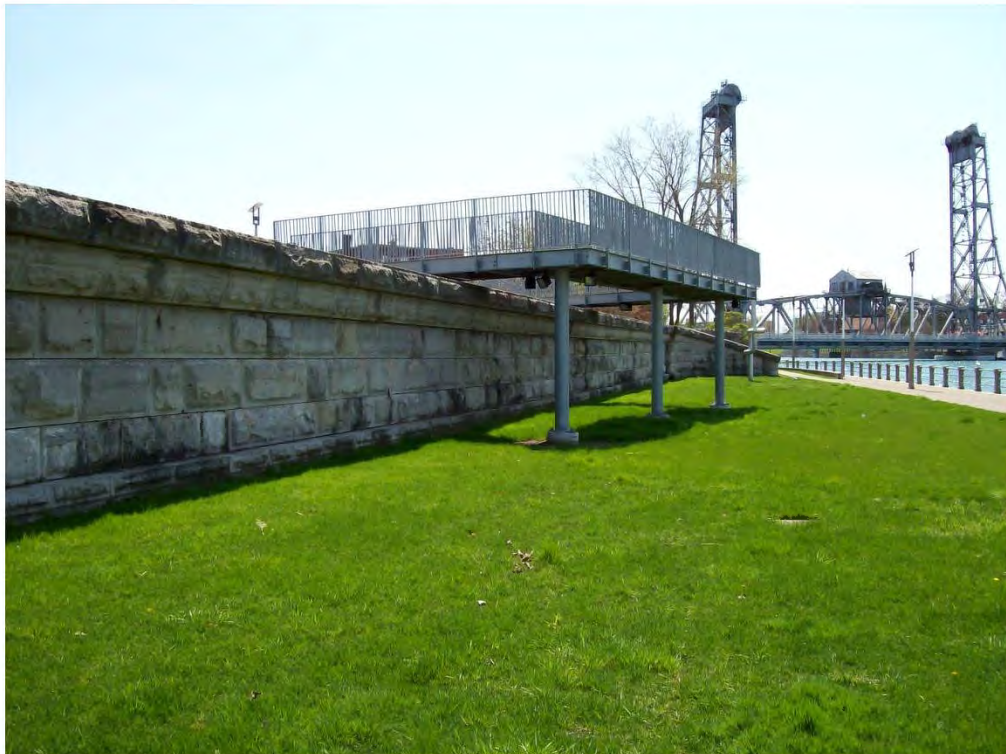
Figs. 13 & 14 Second Canal Aqueduct 2007
