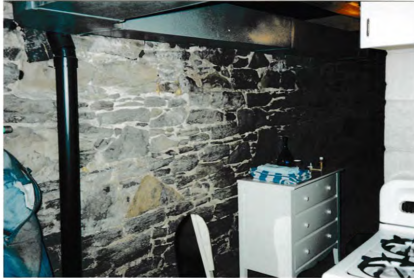
FIGURE 66 Basement - original stone wall and new central block wall (right)
