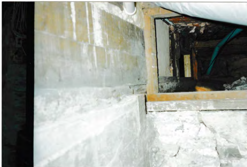
FIGURE 63 Basement crawl space
