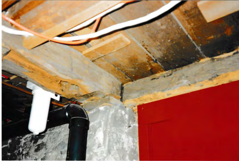
FIGURE 62 Basement ceiling and support beams
