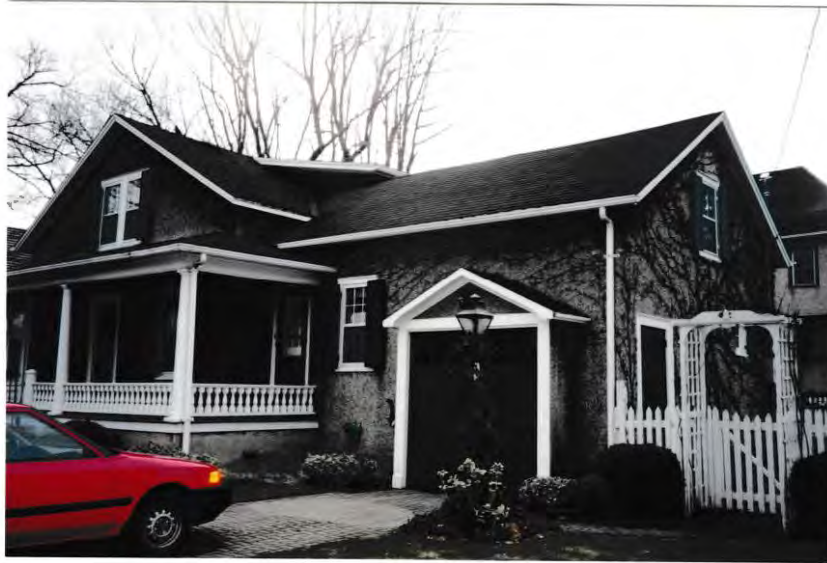
Figure 22 Garage entrance and east end, 1998
