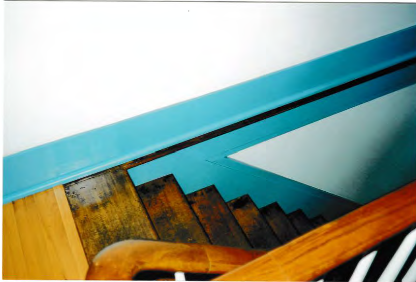
FIGURE 52 Stairs to second floor from front hall. Burn mark from fire visible on fourth step.
