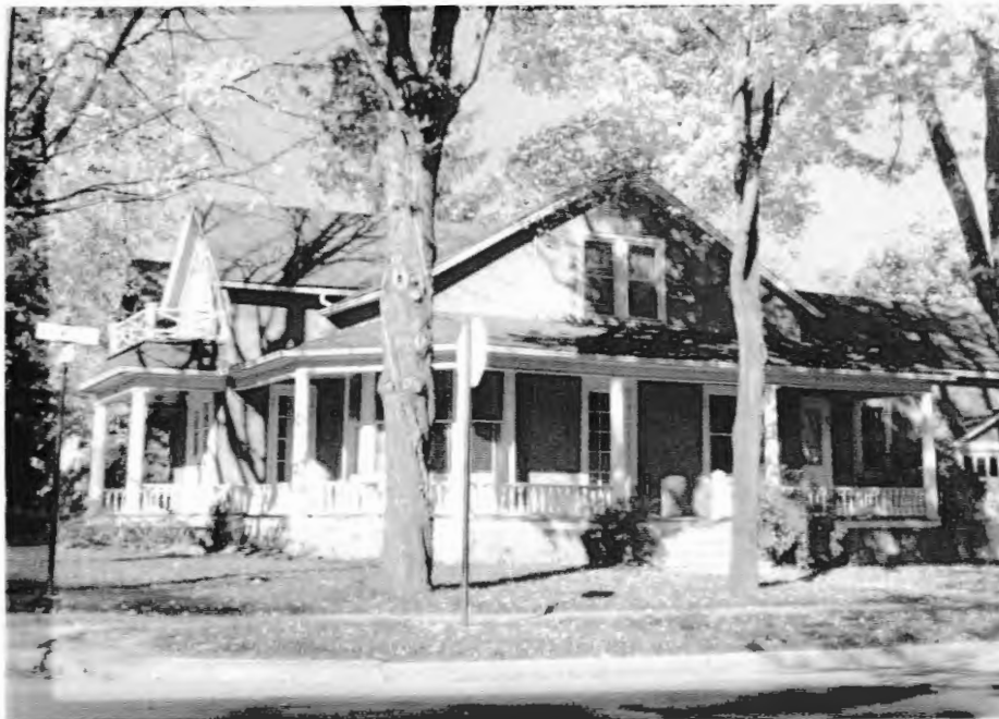
Figure 13 West and south sides, circa 1960's Source: L. Rawlins, F. Devereux
