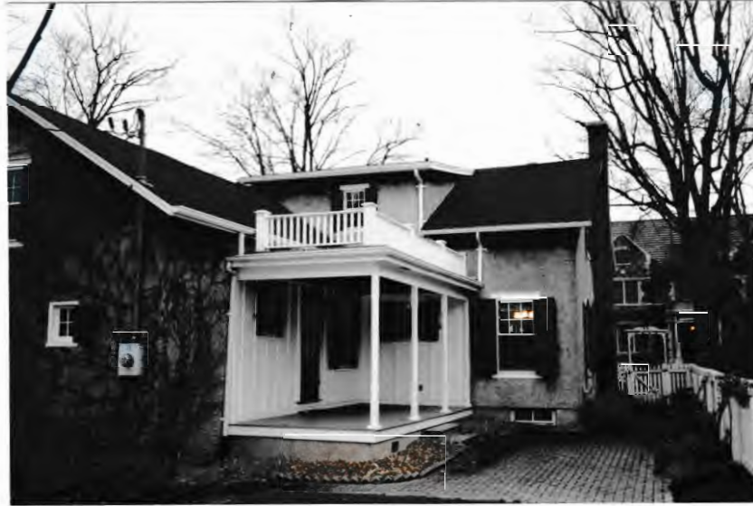
Figure 30 Back porch, north and east walls of house, 1998
