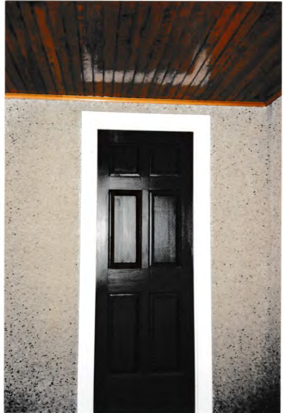
Figure 11 Door under porch and porch ceiling, west side, 1998
