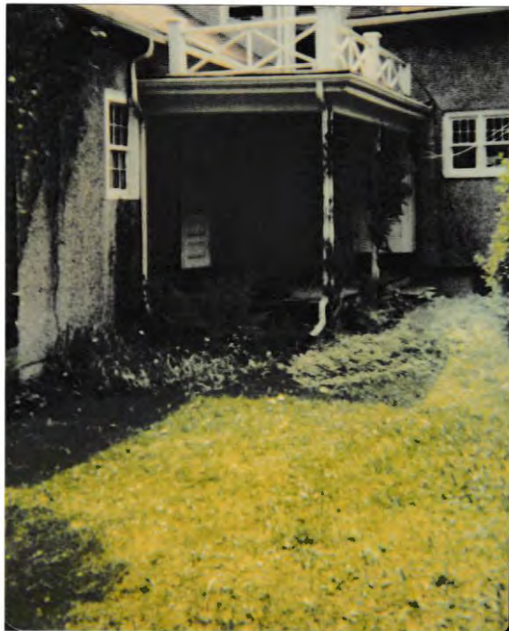
Figures 28 & 29 Back porch, north and east walls of house, circa 1970's. Source: A. Mateka
