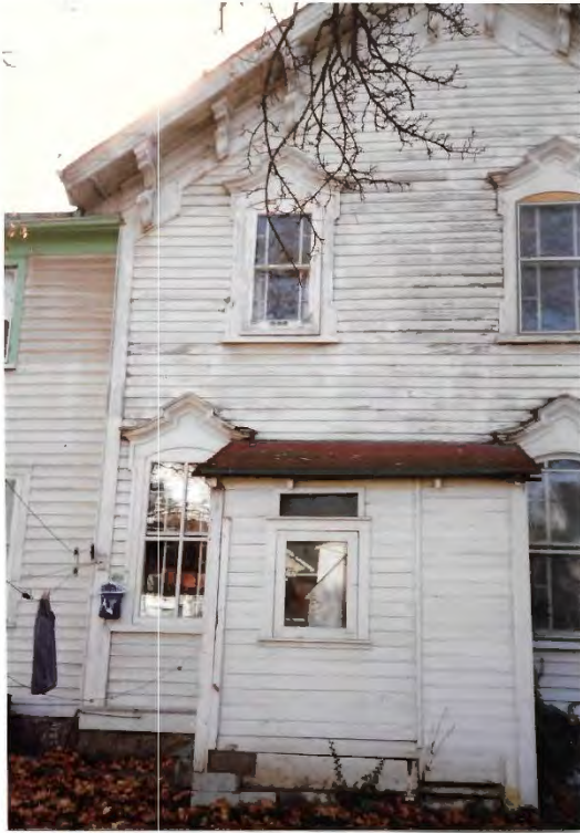
FIGURE 46 WEST WING - NORTH (REAR) FACADE
