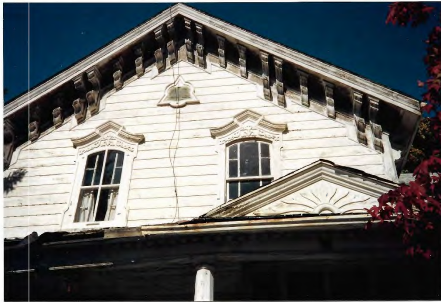
FIGURE 23 WEST WING - EAVES + UPPER WINDOWS
