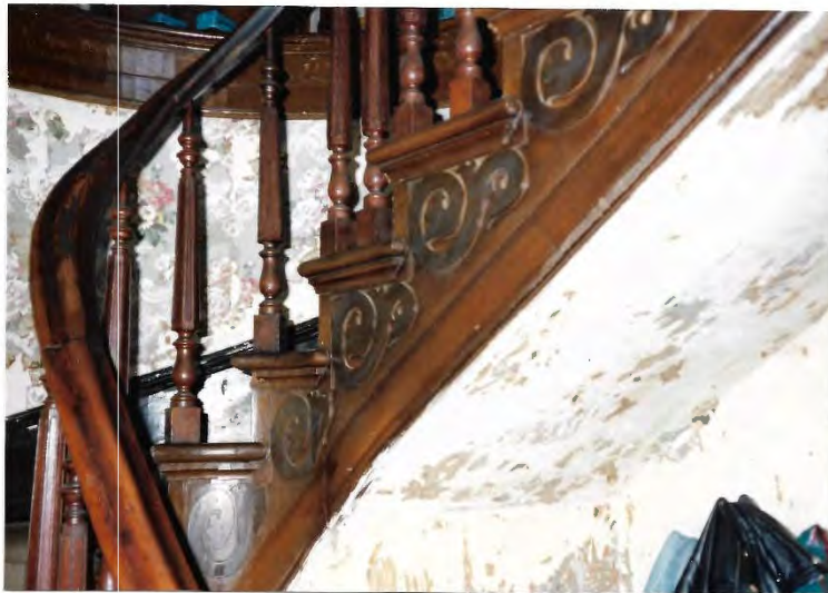
FIGURE 55 FRONT STAIR - WEST WING
