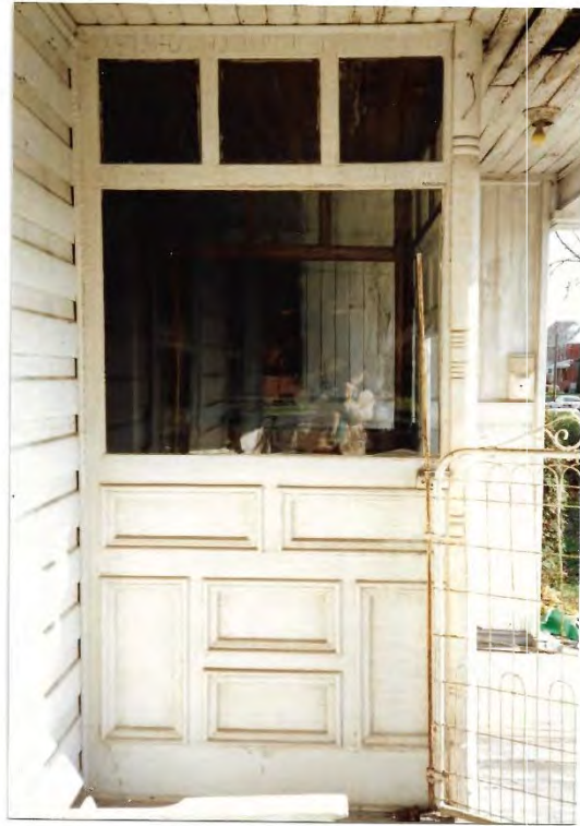
FIGURE 39 FRONT ENTRANCE VESTIBULE -SIDE- WEST WING
