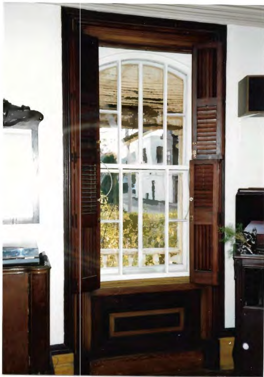
FIGURE 61 FRONT WINDOW - MOULDINGS AND SHUTTERS - LIVING ROOM WEST WING
