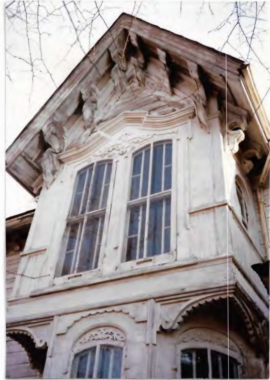
FIGURE 42 BAY WINDOW (UPPER) WEST FACADE
