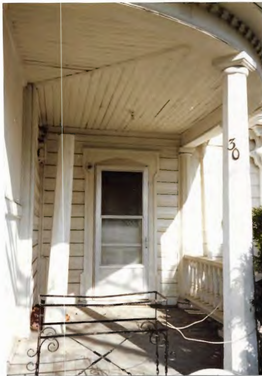
FIGURE 8 FRONT DOOR - EAST WING (EAST END OF FRONT PORCH)
