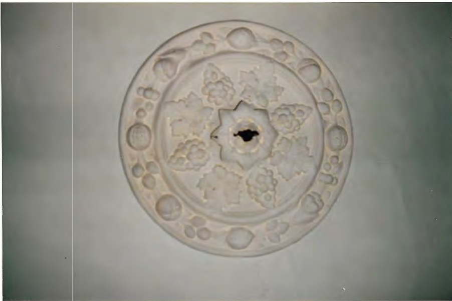
FIGURE 15 CEILING, LIVING ROOM - EAST WING
