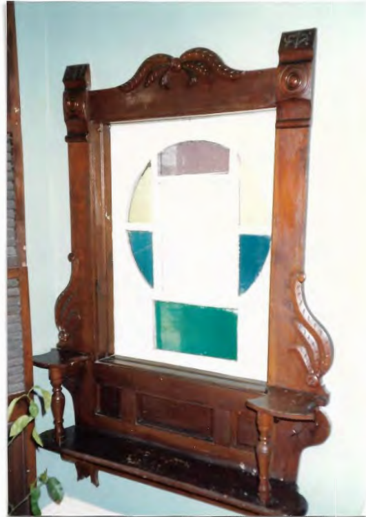
FIG. 73. KEYHOLE WINDOW IN FIG. 72 - BAY, CENTRAL BEDROOM, WEST WING -INTERIOR WITH BUILT- IN SHELF
