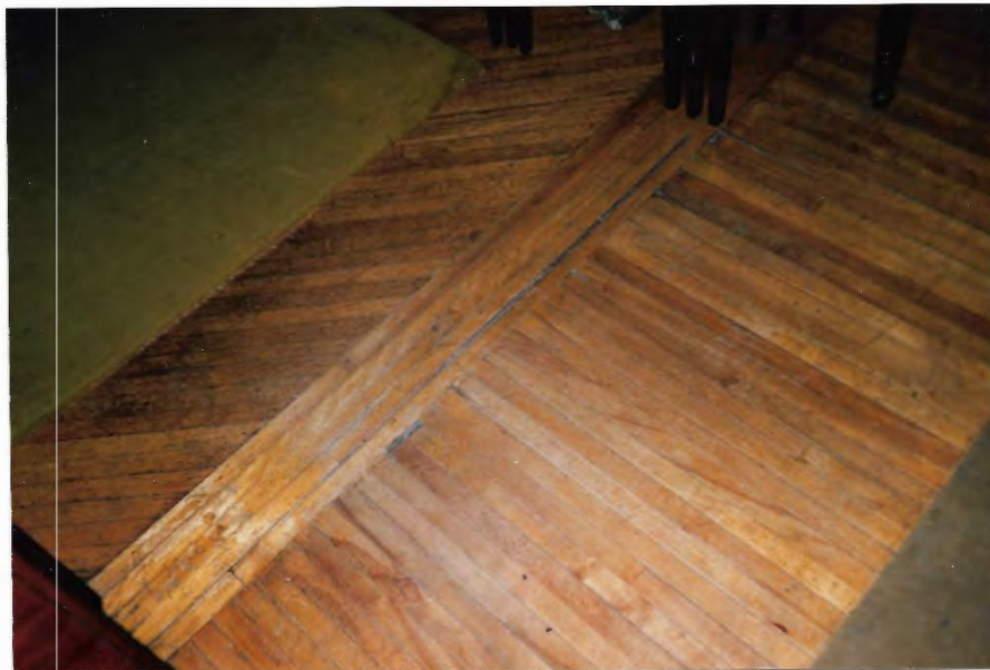
FIGURE 19 HARDWOOD FLOORS - DINING ROOM (RIGHT) LIVING ROOM (DIAGONAL) ON LEFT
