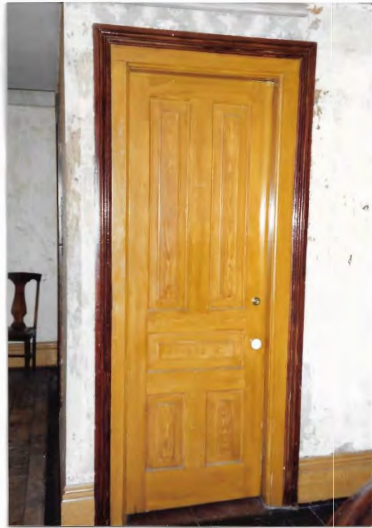
FIG. 70 CLOSET DOOR - UPSTAIRS HALL, WEST WING
