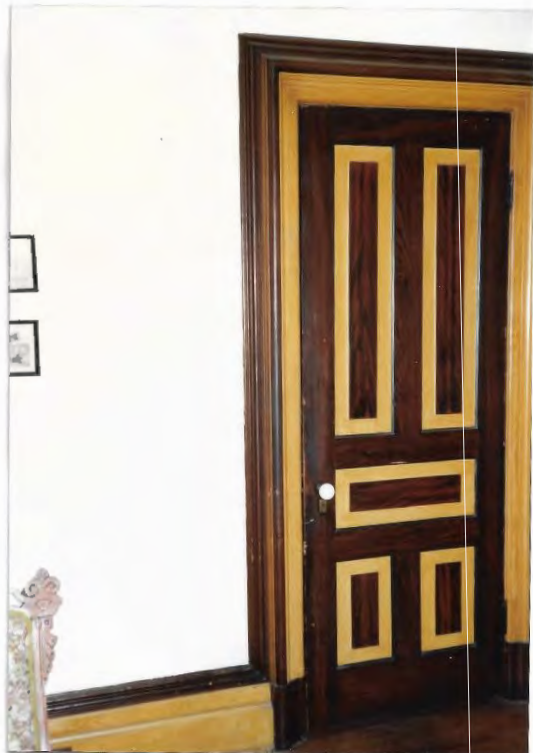
FIGURE 58 DOOR IN FIGURE 57 AND INTERIOR WOODWORK - PAINT GRAINED
