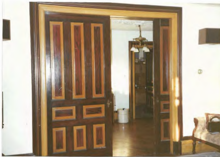
FIGURE 64 SLIDING DOORS BETWEEN LIVING AND DINING ROOMS - PAINT GRAINED WEST WING
