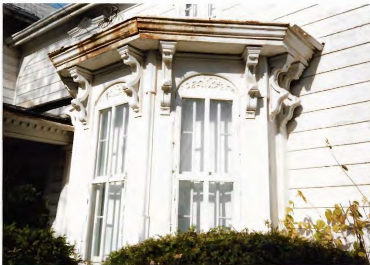
FIGURE 11 EAST WING - BAY WINDOW - FRONT (SOUTH) FACADE
