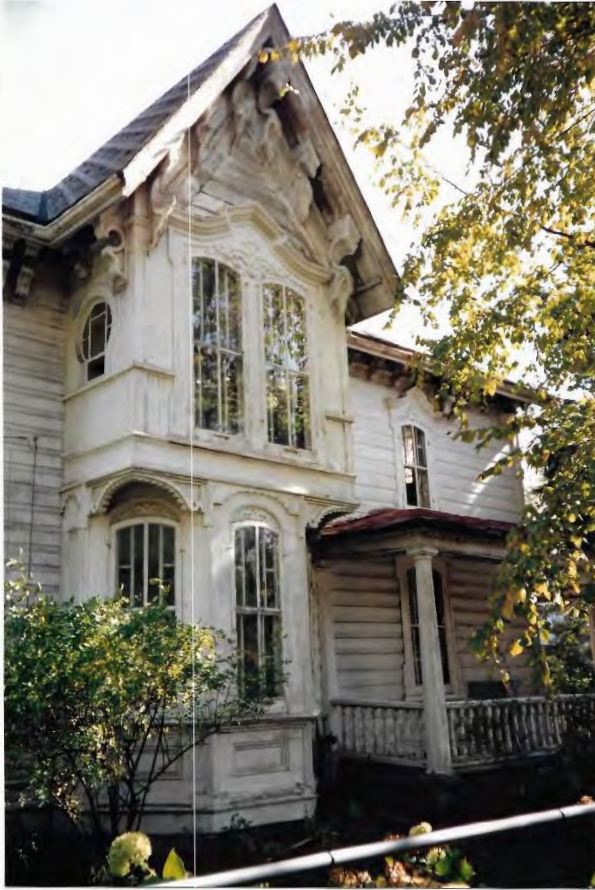
FIGURE 41 WEST FACADE - WEST WING
