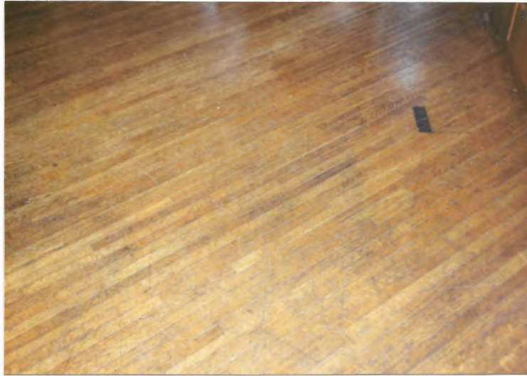
FIGURE 67 DIAGONAL FLOOR (HARDWOOD) IN DINING ROOM, WEST WING
