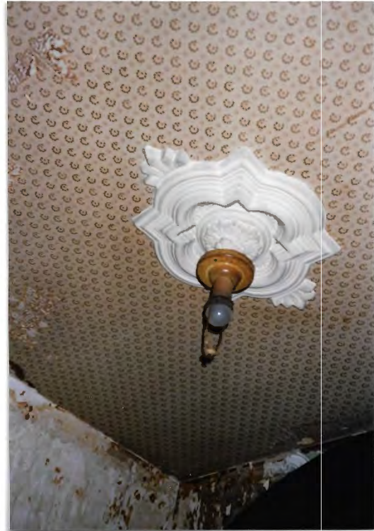
FIGURE 51 LIGHT FIXTURE - FRONT HALL - WEST WING
