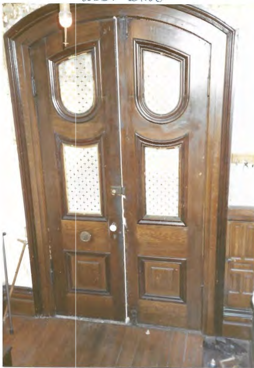
FIGURE 50 FRONT DOOR SHOWING BUILT-IN CUPBOARD (RIGHT)
