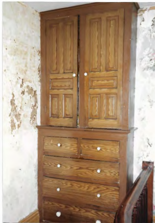
FIG. 71 PAINT GRAINED CUPBOARD UPSTAIRS HALL, EAST WALL - WEST WING
