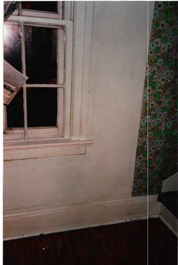
FIGURE 21 EAST WING DINING ROOM WINDOW AND BASE OF STAIRS
