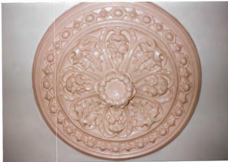
FIGURE 59 MOULDED CEILING DECORATION LIVING ROOM - WEST WING
