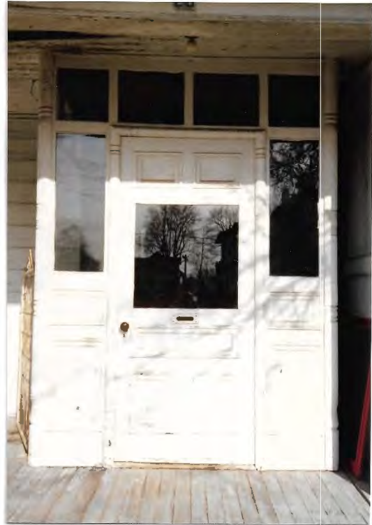
FIGURE 35 FRONT ENTRANCE (WEST WING)
