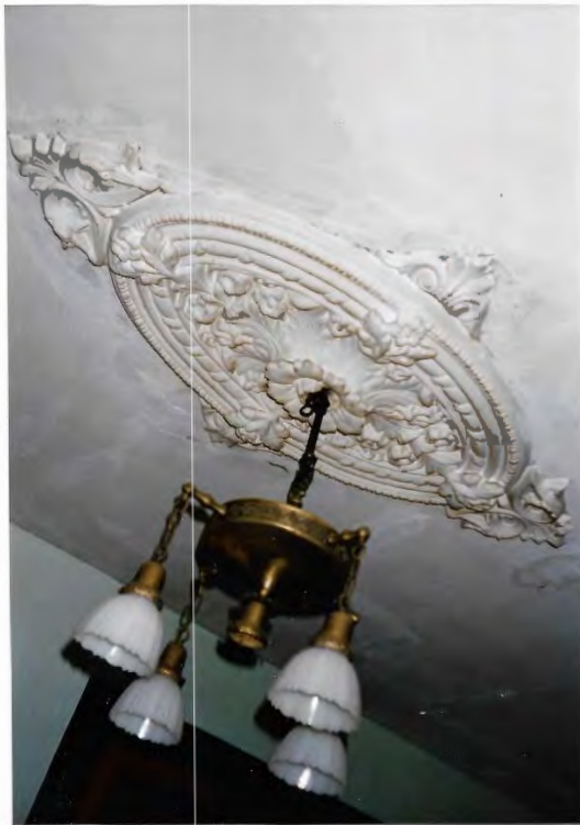
FIGURE 65 ORIGINAL FIXTURE AND MOLDED PLASTER CEILING DECORATION - DINING ROOM WEST WING
