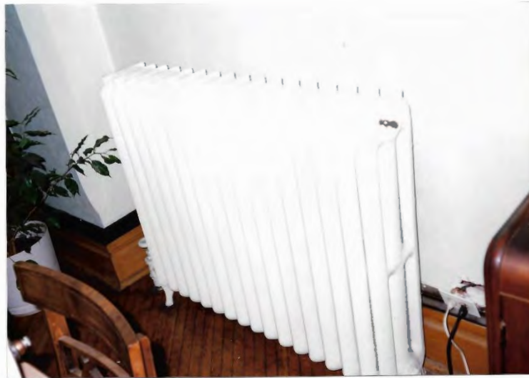
FIGURE 68 PATTERNED RADIATOR DINING ROOM, WEST WING
