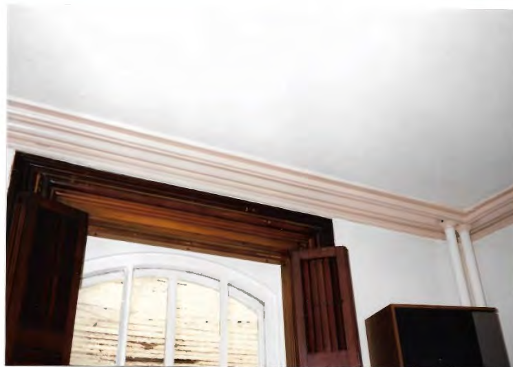
FIGURE 63 CEILING MOULDING AT CORNER LIVING ROOM - WEST WING
