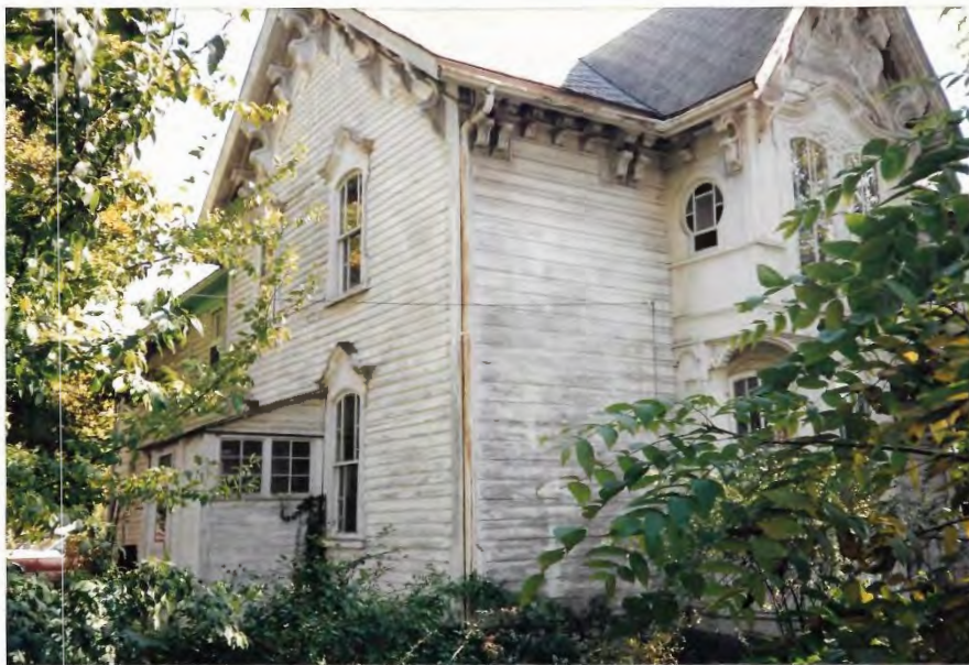
FIGURE 45. MORWOOD HOUSE (WEST WING) FROM NORTH WEST CORNER
