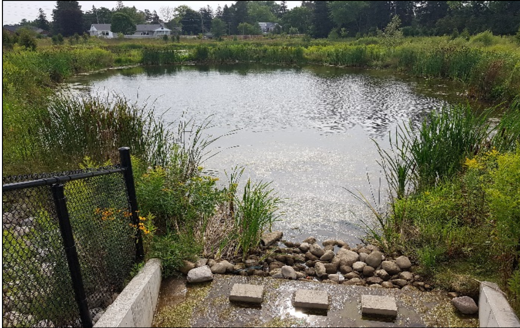
Figure 3-1: A wet pond SWM facility provides water quality treatment via the settlement of suspended pollutants and flood control via the temporary detention and peak flow reduction
