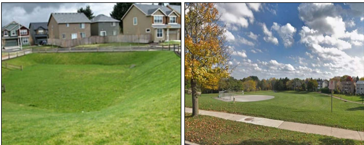
Figure 3-3 – Left: A dry SWM facility provides flood control; but little water quality treatment; Right: A dry SWM facility provides flood control as well as recreational opportunities (Aurora, Ontario)
