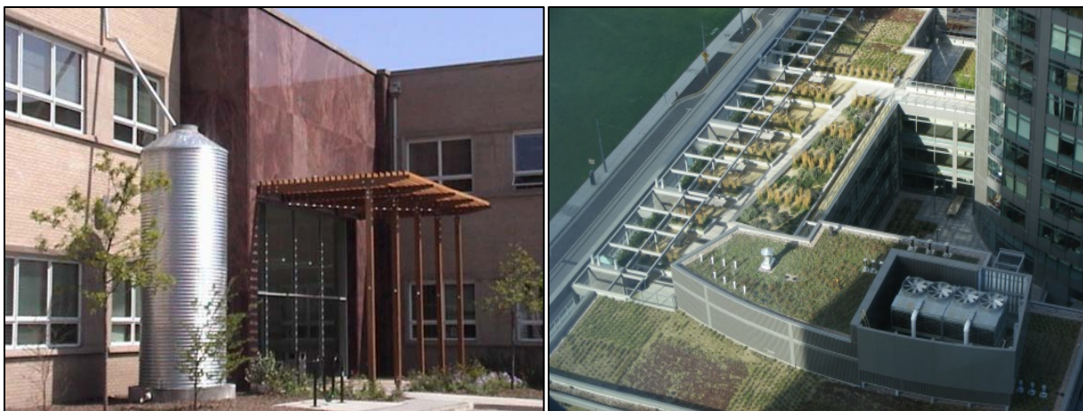
Figure 3-6: Example LID Practices from Left to Right: Green Roofs and Rainwater Harvesting
