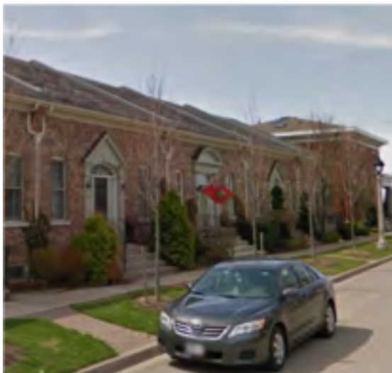
one storey townhomes
