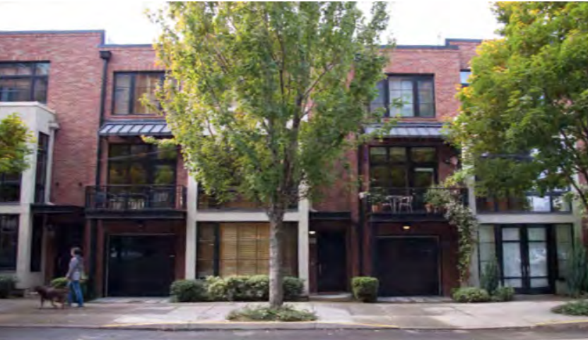
Where front entrance garages are provided, they should be recessed into the building, with built form features above such as balconies that minimize their impact on the public streetscape
