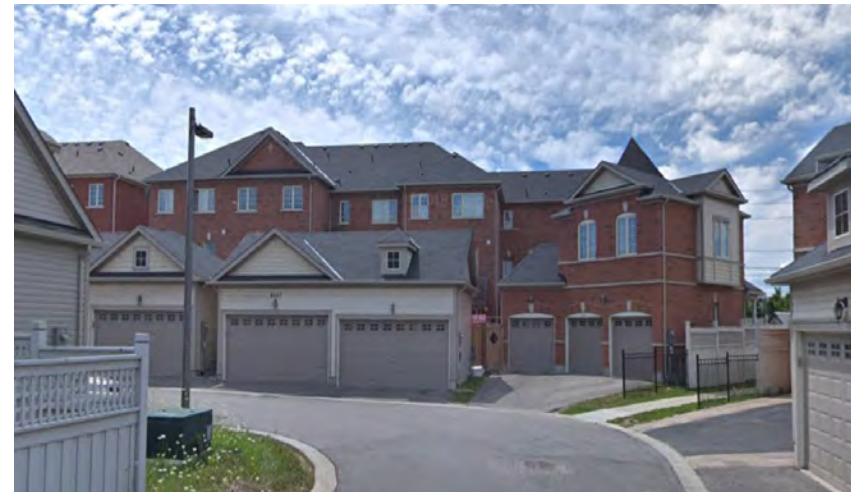
Rear garages should be paired and designed to compliment the main dwelling
