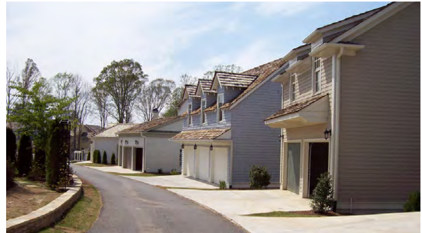
Lane accessed garages help minimize the impact of vehicles within the public realm and should be well articulated to enhance the lane
