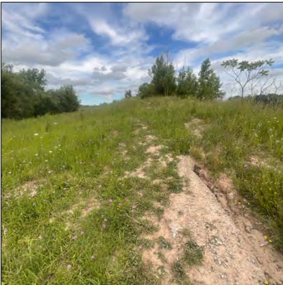
Image 27: Exposed disturbed soils and grading.
