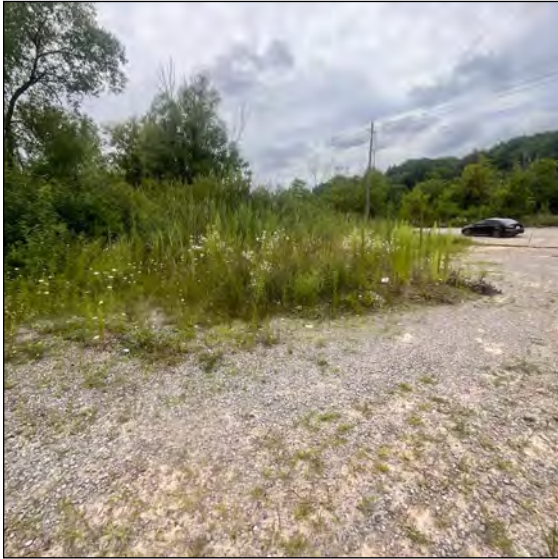
Image 1: Exposed disturbed soils and grading.
