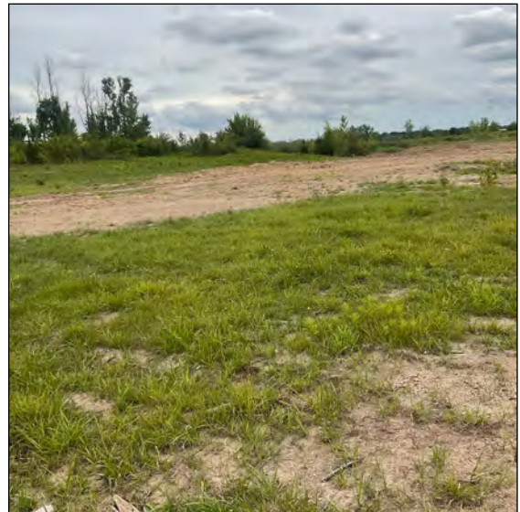
Image 48: Exposed disturbed soils and grading.
