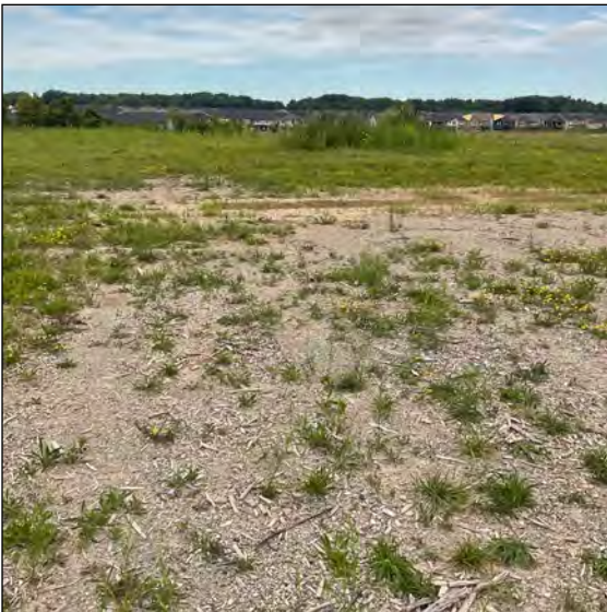
Image 51: Exposed disturbed soils and grading.
