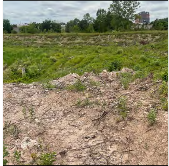
Image 34: Exposed disturbed soils and grading.
