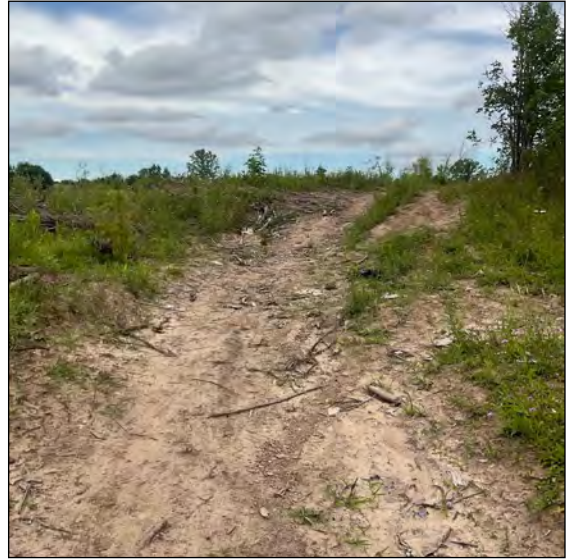
Image 30: Exposed disturbed soils and grading.
