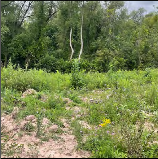
Image 29: Exposed disturbed soils and grading.
