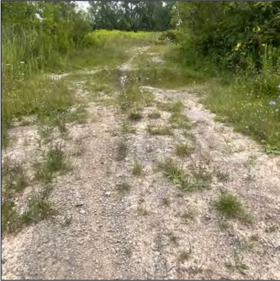
Image 13: Exposed disturbed soils and grading.
