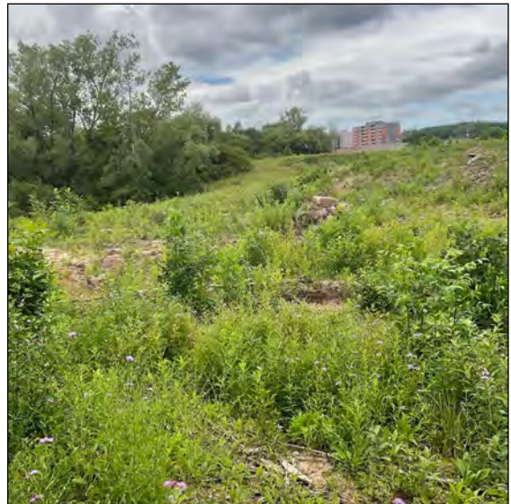
Image 28: Extensive grading and disturbance.
