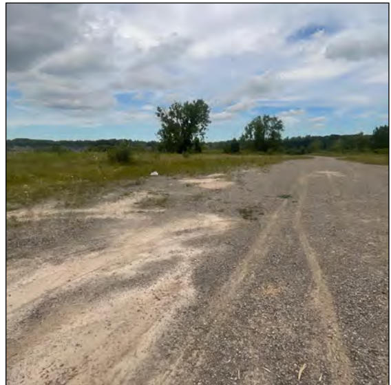
Image 44: Exposed disturbed soils and grading.
