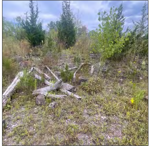
Image 18: Exposed disturbed soils and grading.
